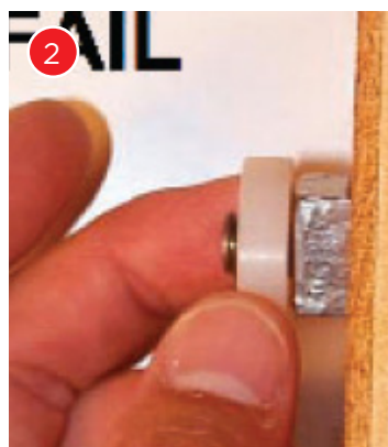
This bolt end is an unsafe protrusion.
